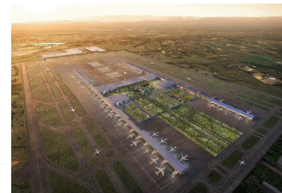
Western Sydney Airport, Australia
